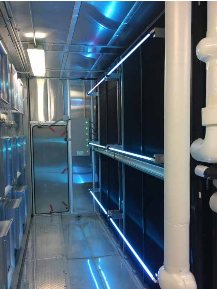
FIGURE 2: UV-C's blue color results from the argon gas in the lamp envelope.
